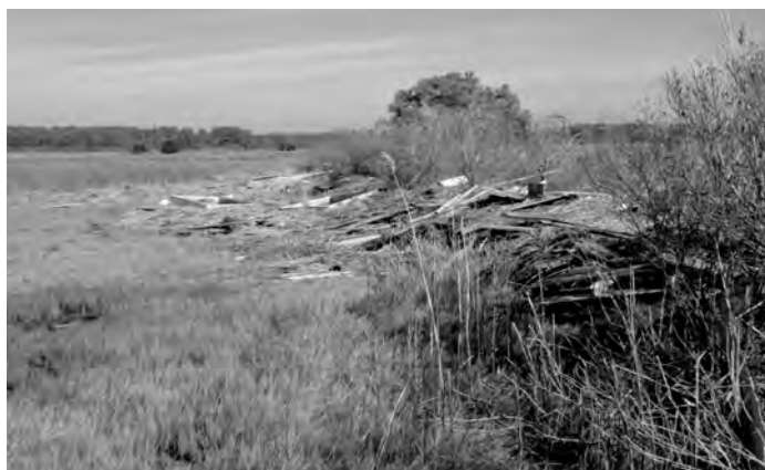
Damage to the Chrisfield tidal dike system by the tidal surge from Hurricane Sandy was assessed and repaired by MDA.
