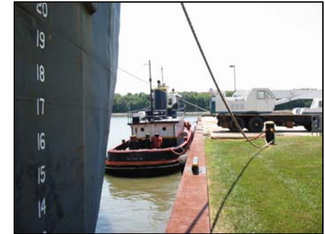
Photo 5.2c Bulkhead – View to Canal
