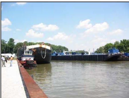
Photo 5.2d Bulkhead – View from Canal
