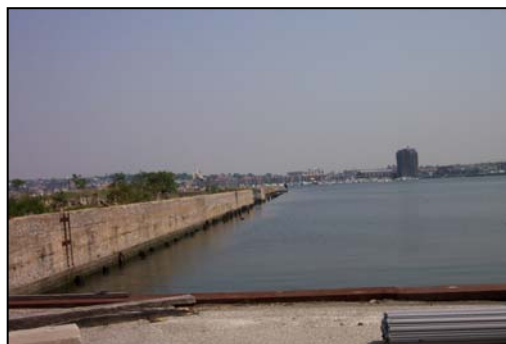
Photo 5.3e Bulkhead – View to Pier 8
