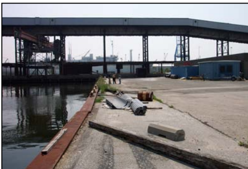
Photo 5.3d Bulkhead – View to Pier 7
