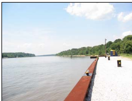
Photo 5.2e Canal Bulkhead–View to Bay
