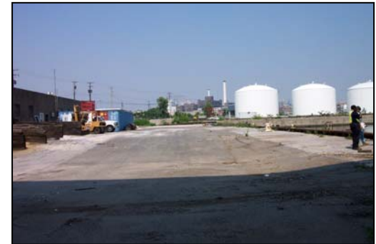
Photo 5.3c Waterfront Access Road
