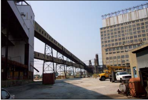
Photo 5.3a Pier 7 Access Driveway
