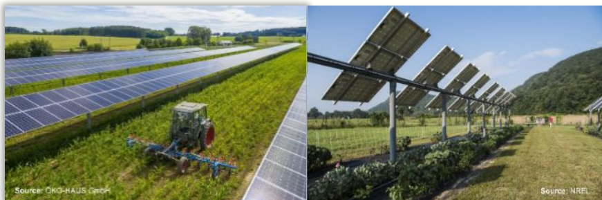
Figure 2. Agrivoltaic examples with elevated racking and optimized row spacing to accommodate farm machinery and field operations.
