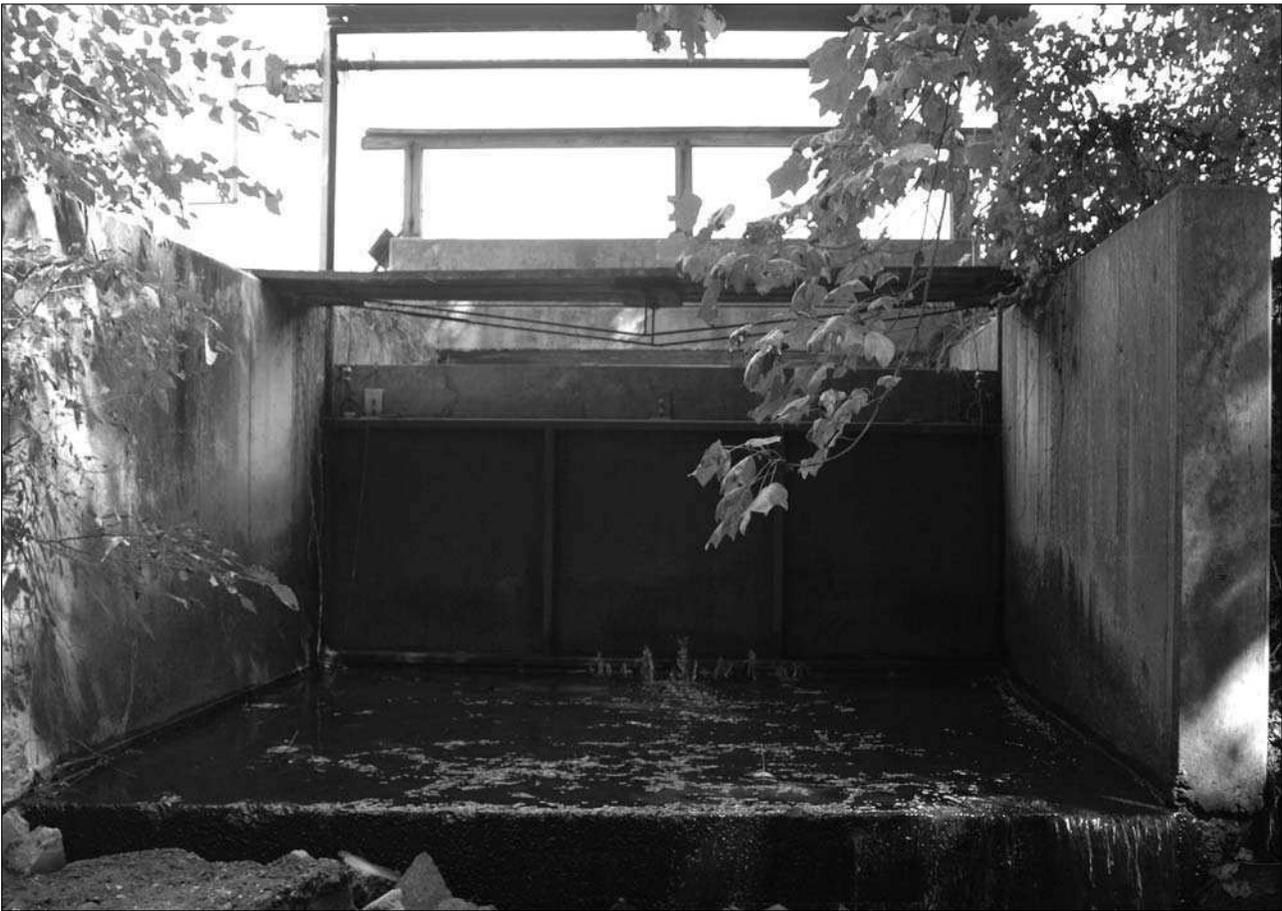
Dam board riser systems such as this one allow regulation of water depth in ponds, a cost-effective measure for controlling pond weeds. These structures can lower water levels to dessicate shallow vegetation, for example, or raise levels during periods of high flow to float weeds downstream.
