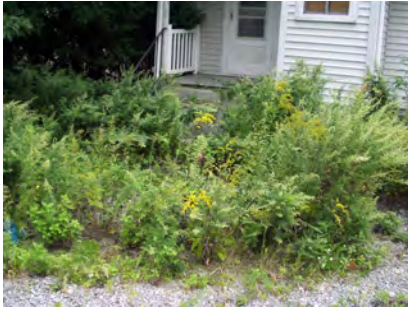
Weeds and plants along foundations provide rodents with hiding places, nesting sites, and hidden runways, while also making the area difficult to inspect. (Photo L. Pinto)
