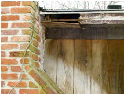
Roof rats often enter buildings through openings at or near the roof. (Photo L. Pinto)
