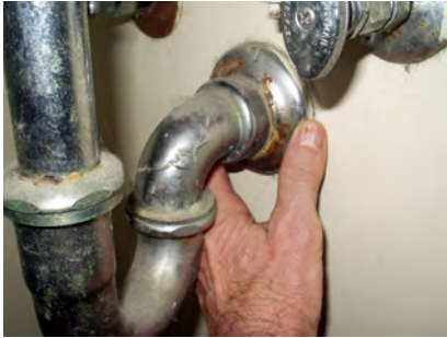
Escutcheon plates can be installed around utility lines to prevent rodents from moving in and out of wall voids. (Photo L. Pinto)
