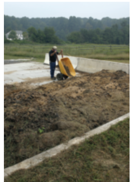
Manure storage structure with Jersey walls and concrete floor.
