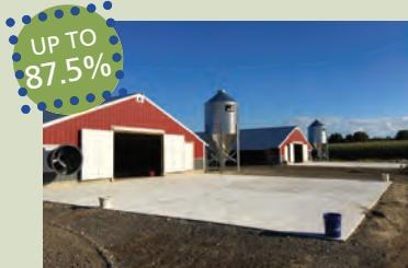
**HEAVY USE AREA PADS** can be installed at poultry house entrances to protect against runoff during cleanouts.
