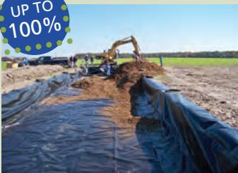
**SUBSURFACE DENITRIFYING BIOREACTORS** are trenches filled with a carbon source—usually wood chips—and installed at the edge of a field to remove nitrate nitrogen from agricultural drainage water.
