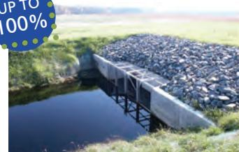
**GRADE STABILIZATION STRUCTURES** can be used at the outlet of a grassed waterway to help prevent gully erosion.
