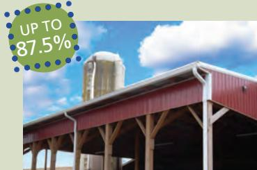
**ROOFS AND COVERS** can be installed over an existing or planned heavy use area to help divert clean water away from barnyards and feedlots.
