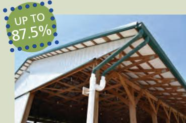
**ROOF RUNOFF STRUCTURES** are gutters, downspouts and outlets that can be installed on farm buildings to prevent rainwater runoff from mixing with manure.
