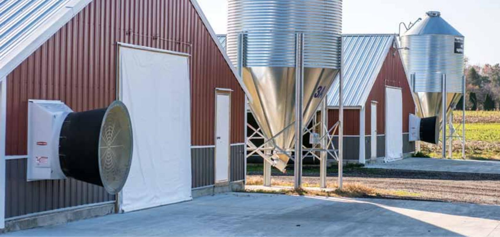
A CONCRETE PAD CONSTRUCTED AT THE ENTRANCE TO A POULTRY HOUSE IN QUEEN ANNE'S COUNTY HELPS PROTECT GROUNDWATER AND SURFACE WATER DURING CLEANOUTS.
