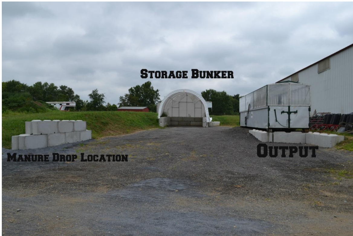
Figure 2. Earth Flow compost unit, storage/curing bunker, and manure drop.
