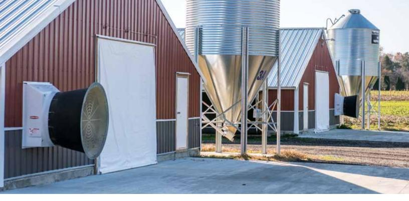
A CONCRETE PAD CONSTRUCTED AT THE ENTRANCE TO A POULTRY HOUSE IN QUEEN ANNE'S COUNTY HELPS PROTECT GROUNDWATER AND SURFACE WATER DURING CLEANOUTS.
