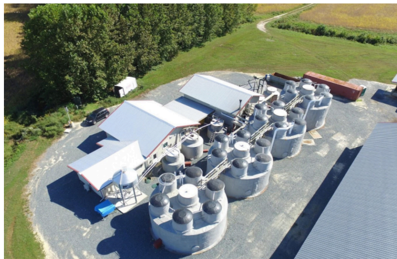
Figure 1. Planet Found Energy Development's anaerobic digestion and nutrient capture system at Millennium Farm. Credit: PFED.
